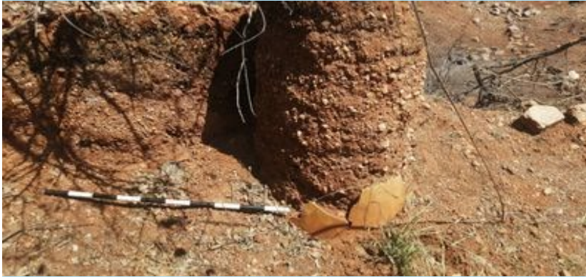
Figure 7-45: A column of the homestead with bits of thin concrete attached
