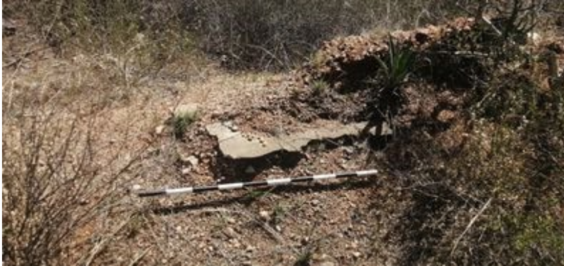
Figure 7-40: Portions of concrete flooring still preserved
