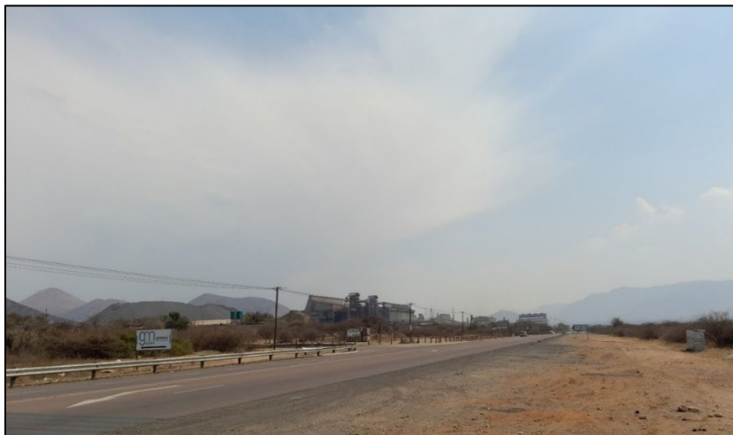
Figure 4 - The Tubatse Ferrochrome Smelter as viewed from the R555 road to the north-east of the Smelter.
