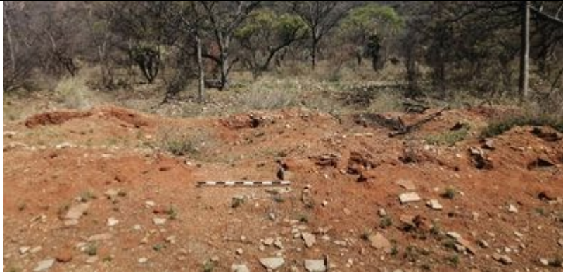
Figure 42 – Poorly preserved historic homestead. Made of mud, stone and cement. Only foundation with bits of crumbled walling have preserved.
