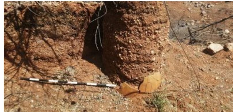
Figure 57 – A column of the homestead with bits of thin concrete attached.
