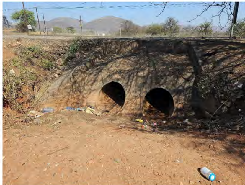
Figure 6-9: R555 double barrel culvert system
